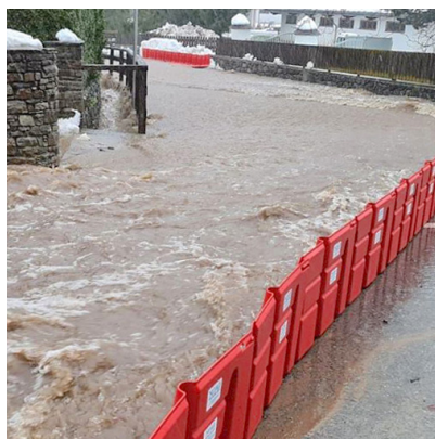
Several BW52 boxes built as a wall can hold back floodwater
