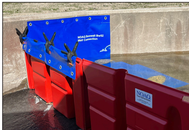
The NOAQ Wall Connector hung against the wall with hooks in the eyelets and attached to the box with clamps
